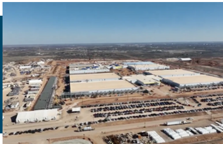
Aerial view of ongoing construction of the first phase of The Stargate Project in Abilene, Texas, a collaboration of OpenAI, Oracle and Softbank. Credit: OpenAI
