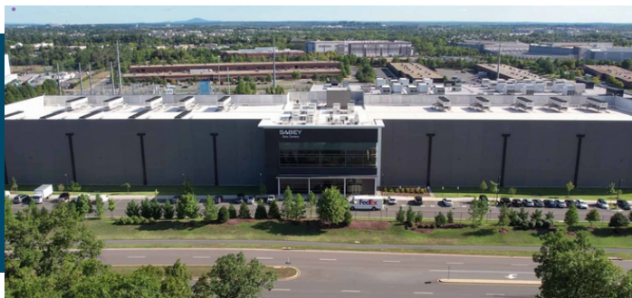
One of numerous Sabey Data Centres located in the heart of Data Center Alley. Credit: Sabey Corp.
